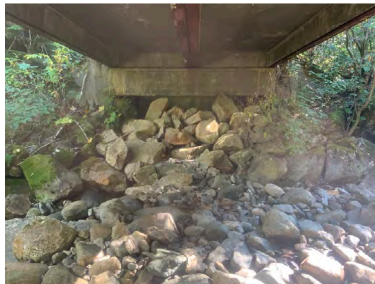
Right Bank Abutment when facing downstream
