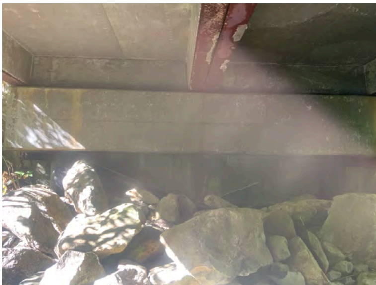
Left Bank Abutment when facing downstream
