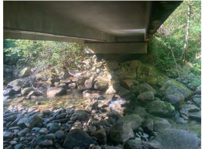
Left Bank Abutment when facing downstream
