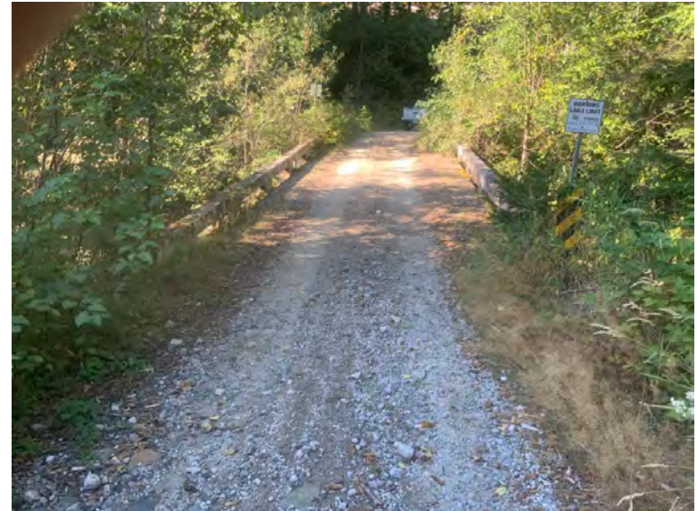
Right Bank Abutment when facing downstream
