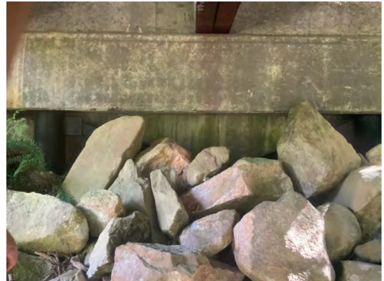
Right Bank Abutment when facing downstream
